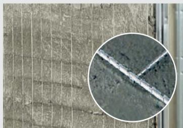
Cement plastering does not fall because it is hold by the knurled thick mesh\* (25 x 50 mm) placed in between the plate and the edge of the cement plastering.
